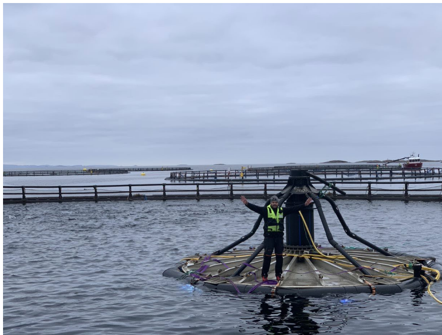
Figur 6 Luft kuppel under montering
